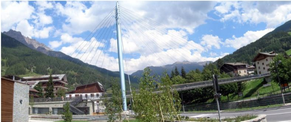
Figure 2: A view of the Bormio footbridge
