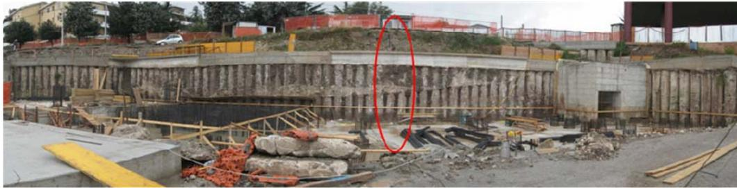
Figure 1: View of the flexible retaining wall and of monitored pile location.
