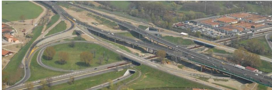
Figure 3: Aerial view of the new viaducts over Forlanini Avenue, Milan, Italy. (Courtesy of G. Massone and G. Pasqualato, Sineco S.p.A.)
