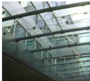
Figure 4: Glass truss of the restaurant of the Zwitserleven building in Amstelveen.
