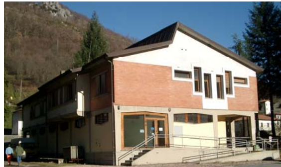
Figure 1: General view of the building.
