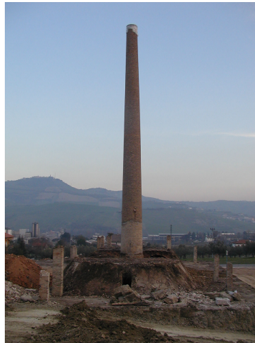
Figure 1: The masonry chimney.
