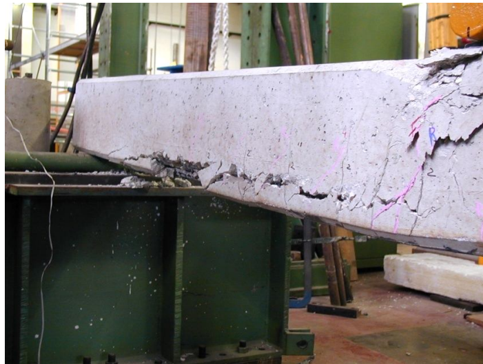
Figure 10: Failure view of strengthened RC beam (B2)
