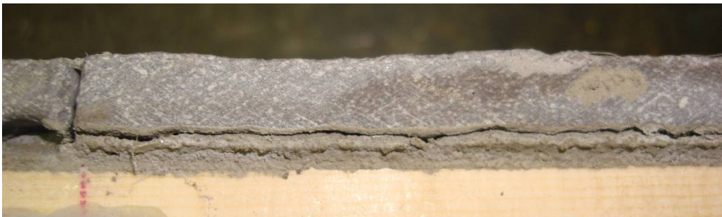
Figure 13: Cracking of the adhesive along an horizontal line.
